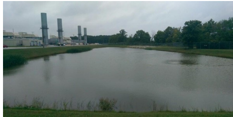
Troy Energy plant, formerly owned by GDF
